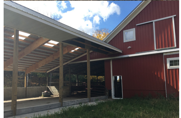
Heavy use area before (top) and after (bottom) implementation of a heavy use area protection BMP. This project reduced erosion and surface runoff of agricultural waste.
