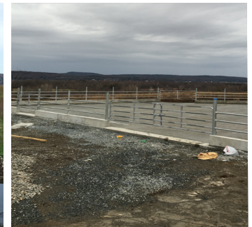
Before (left) and after (right) installation of a Heavy Use Protection practice to address runoff and erosion risks
